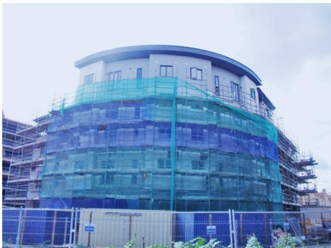
The timber frame six-storey C block, including 8 2-bed flats, and complex radius interior and exterior walls, nears completion.
